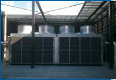
▲ The centrepiece of the concept: JAEGGI Hybridtechnologie AG's hybrid dry coolers
