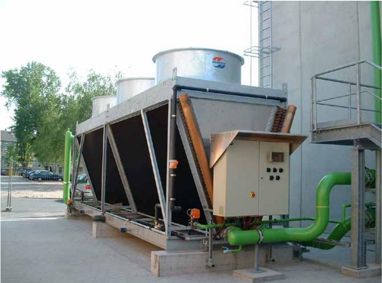
Hybrid dry cooler HTK 2.4/9.0 for cooling a test facility, cooling capacity 1,900 kW at fluid temperatures of 35/28 °C, Photo: JAEGGI Hybridtechnologie AG
