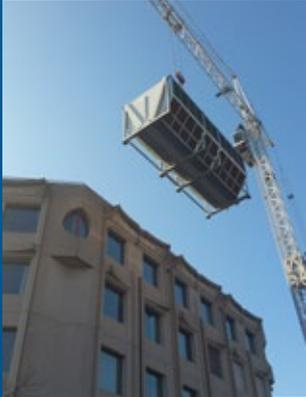
▲ A crane lifts a 4,600 kg JAEGGI adiabatic cooler onto the roof of the office building of DuPont de Nemours.
