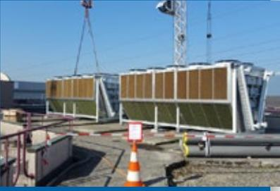
▲ ...and replaced by space-saving JAEGGI ADC adiabatic coolers.
